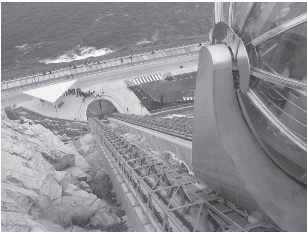
Inclined elevator A Coruña
